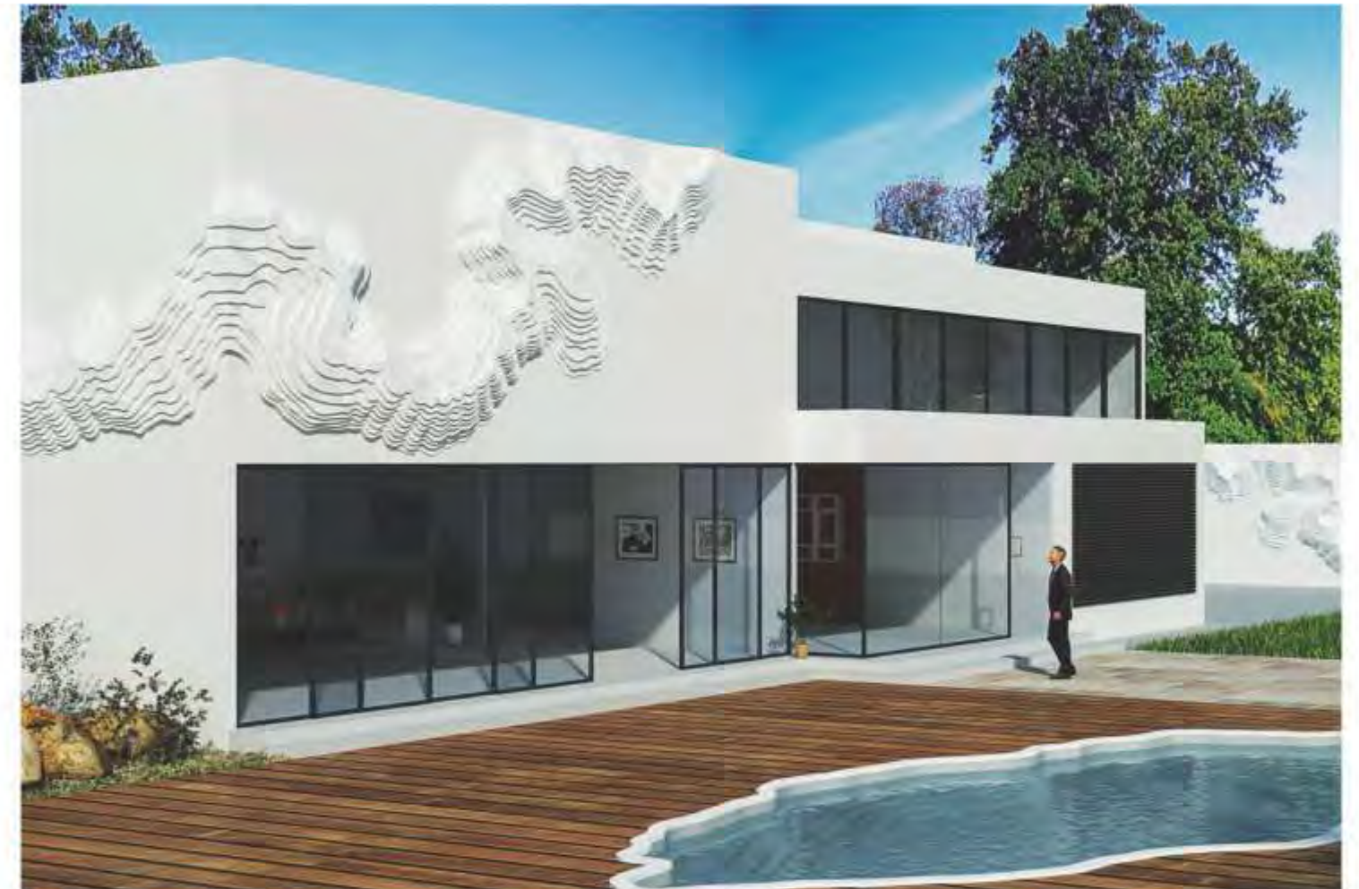
ABOVE | Topographie wrapped around the Facia & Boundary Wall of the project
