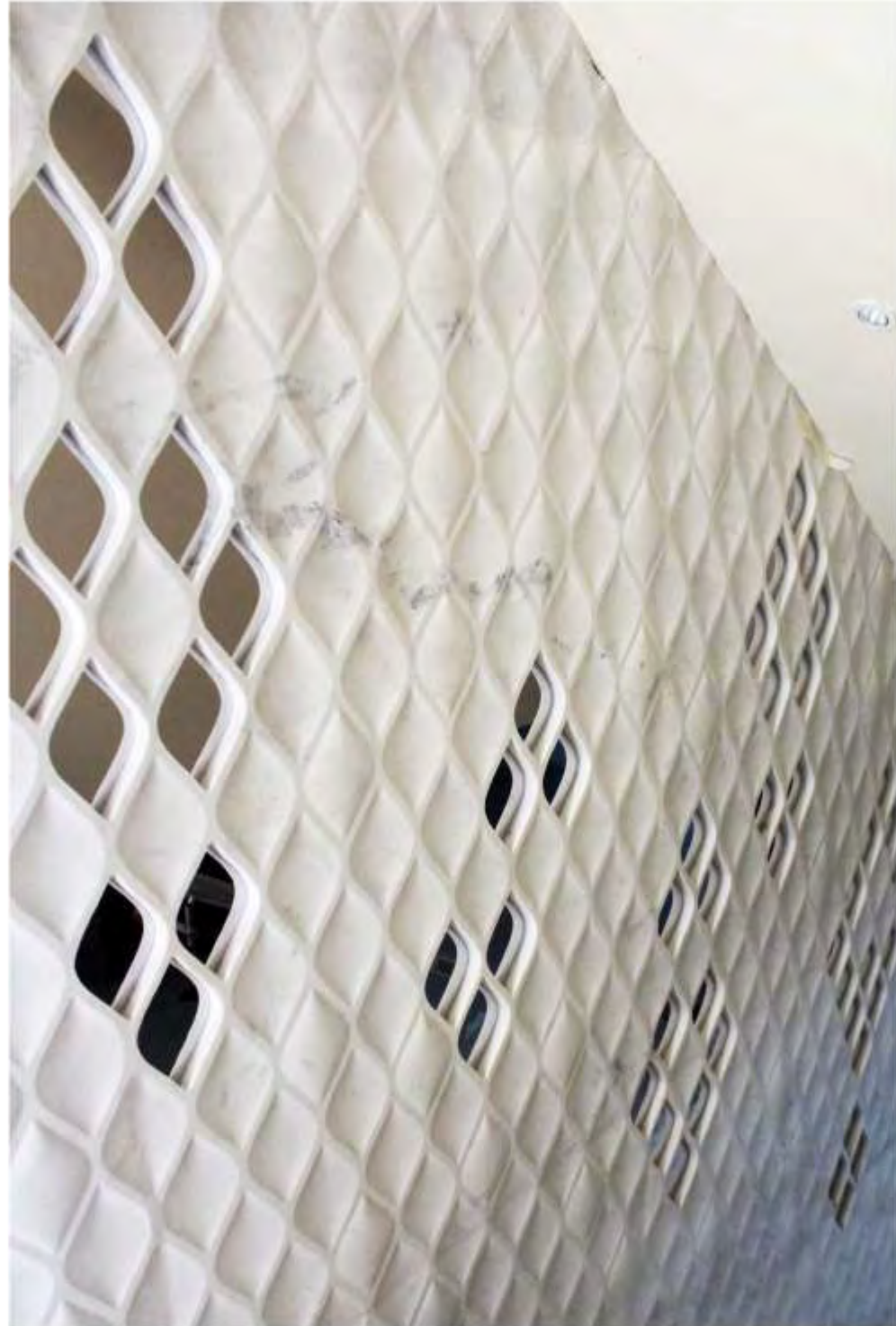
ABOVE AND RIGHT | Dewdrop Staircase with Jaali and It is Backed with SS Sheet
